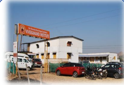
VIVEKANAND INSTITUTE Pegalwadi Trimbakeshwar -a 18000 sq.ft infrastructure with ultra modern facilities for better learning
